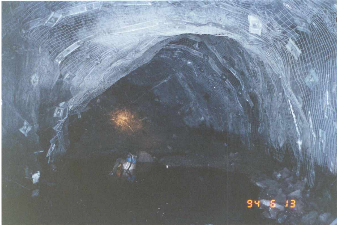
Bursting from back and walls in Dolerite (obviously meshed)
